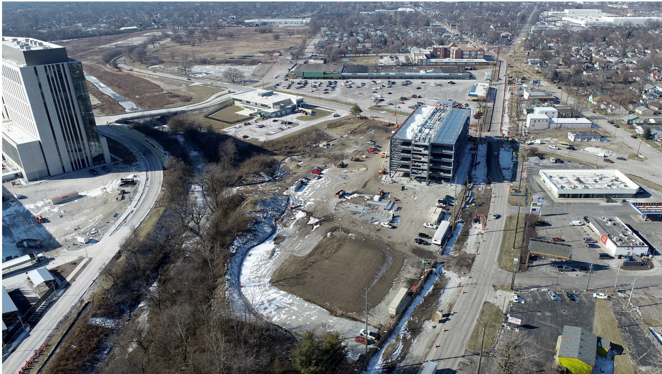
Aerial – looking West
