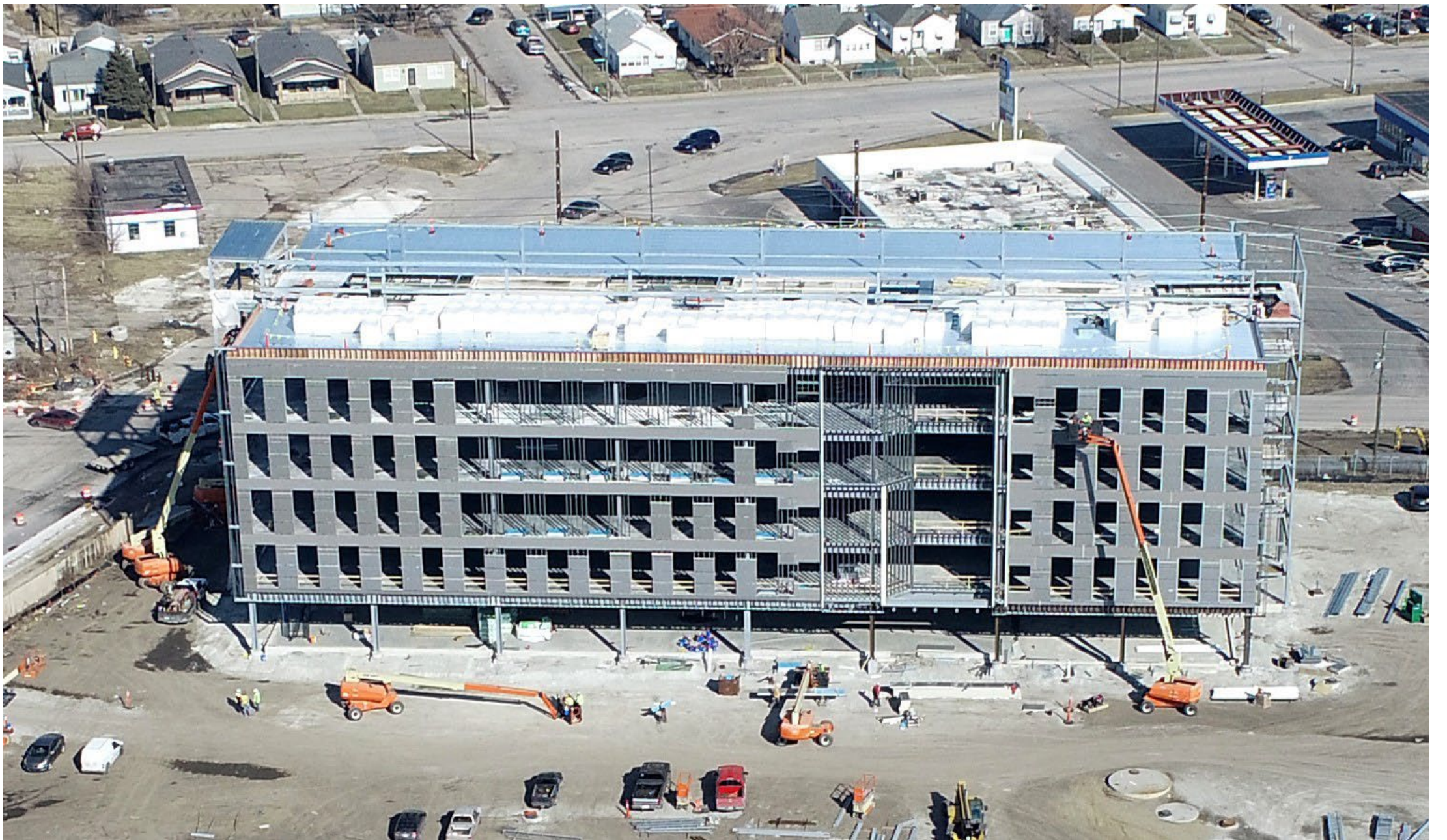
Close up aerial – looking North
